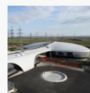
Power Grid Control Centre Read more...
